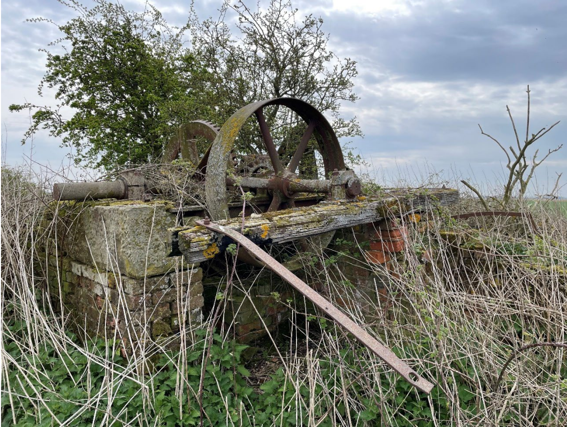
Closer view of drainage pump, looking south-east
