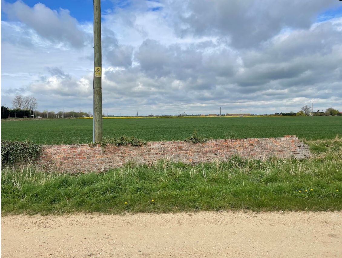
Close-up view of brick walling
