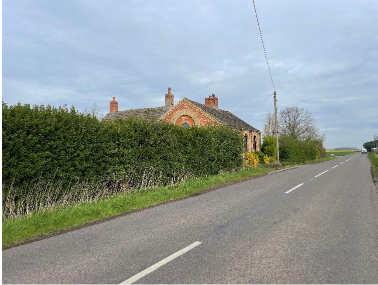
Plate 25: View of former Primitive Methodist Chapel from Sidebar Lane, looking north
