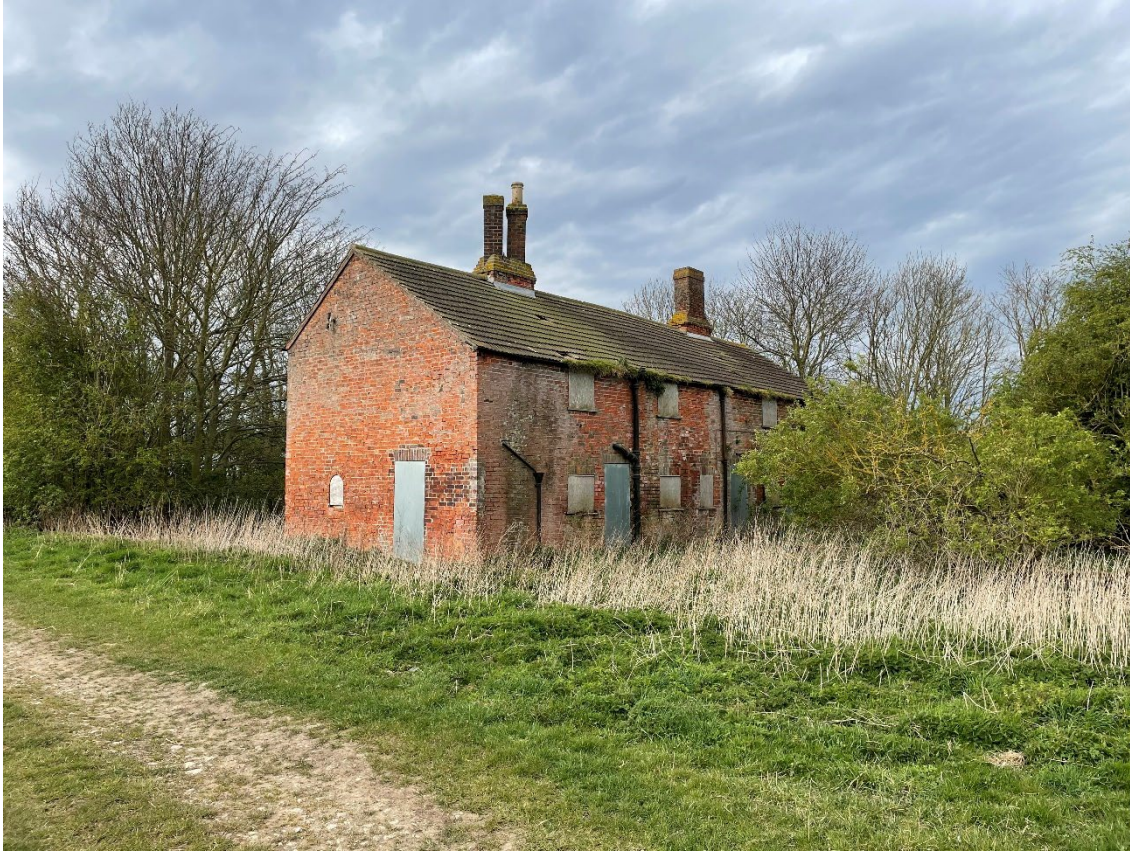
East- and north-facing elevations of the cottage(s) at Six Hundreds Farm
