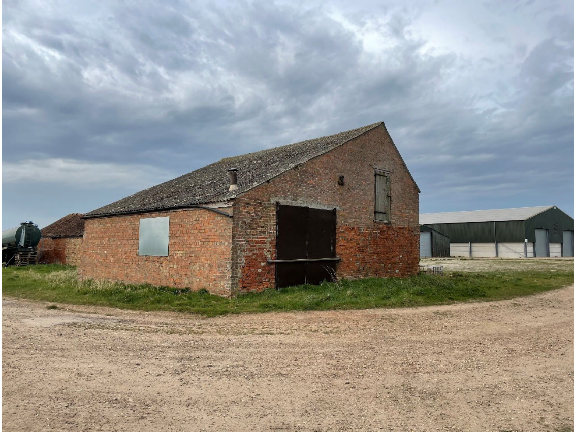
East and north-facing elevations of the northernmost of the two barns at Six Hundreds Farm
