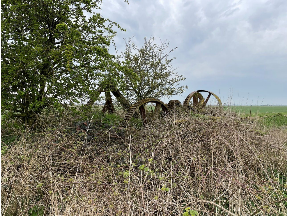
Remains of drainage pump, looking south
