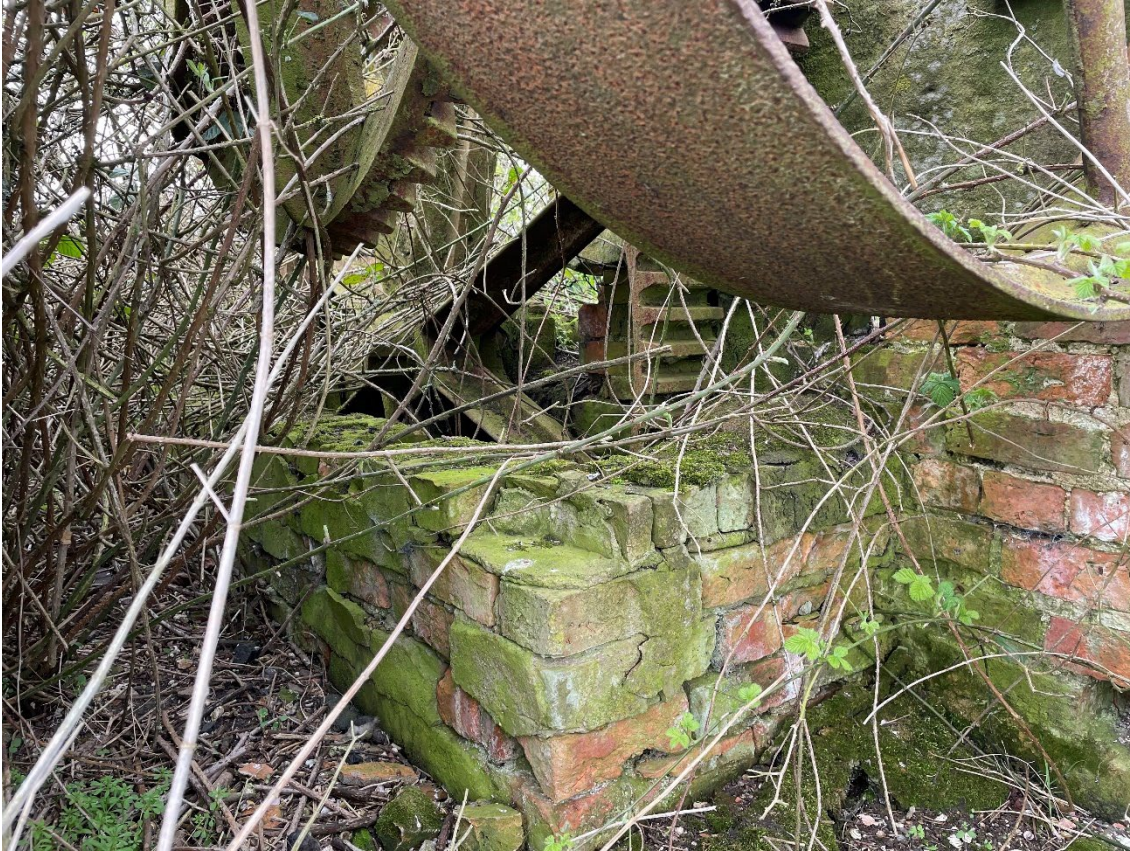
Close-up view of brick base
