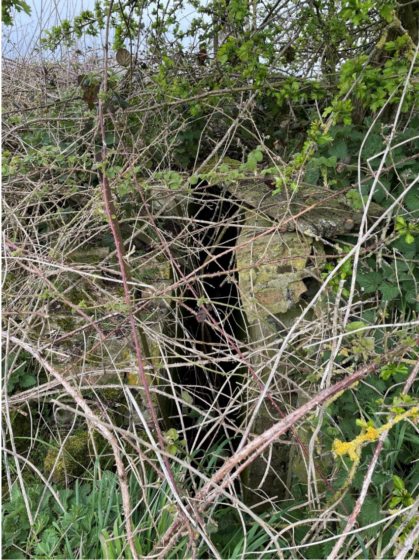
Close up view of brick channel walls, looking west
