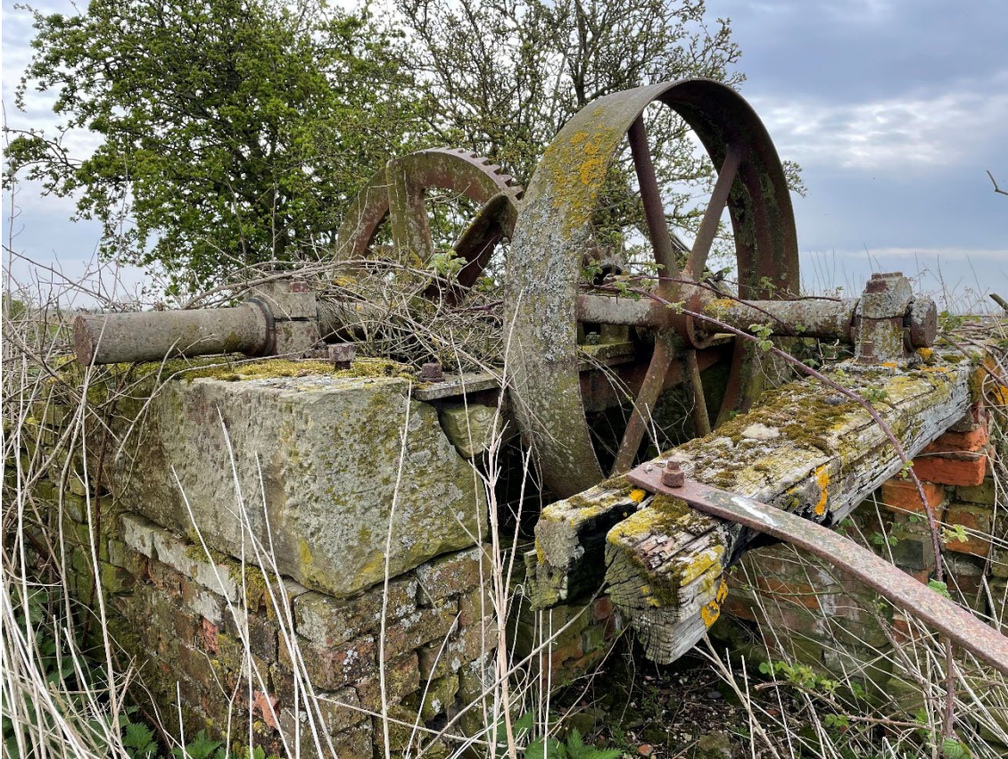
Close-up view of the cast iron scoop wheel on gritstone mounting block above brick base
