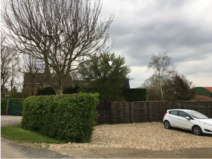
Plate 16: Glimpse of the Drainage Mill at Spinney Farm
