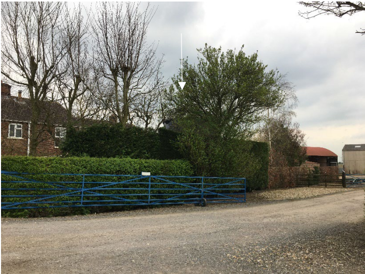
Plate 15: Glimpse of the Drainage Mill at Spinney Farm
