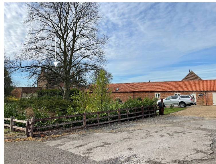
Plate 12: View of Bridge House (arrow) from the barns' private access off the A17
